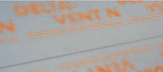
Product identification markings serve as a guide for overlap edge.
