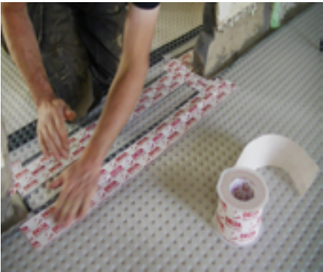
28. Applicera DELTA®-MULTIBAND runt om. Applicera DELTA®-MULTIBAND runt om.
