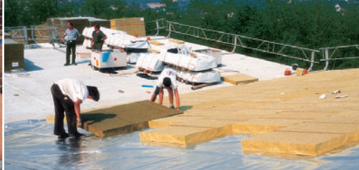
Typical application on lightweight industrial roof.
