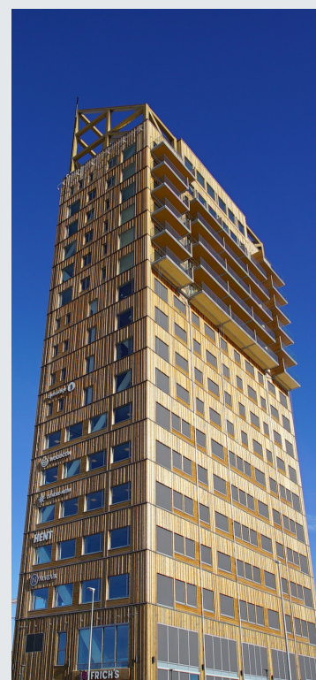
Facts: Exterior cladding of Thermowood-D impregnated with Woodsafe Exterior WFX.
