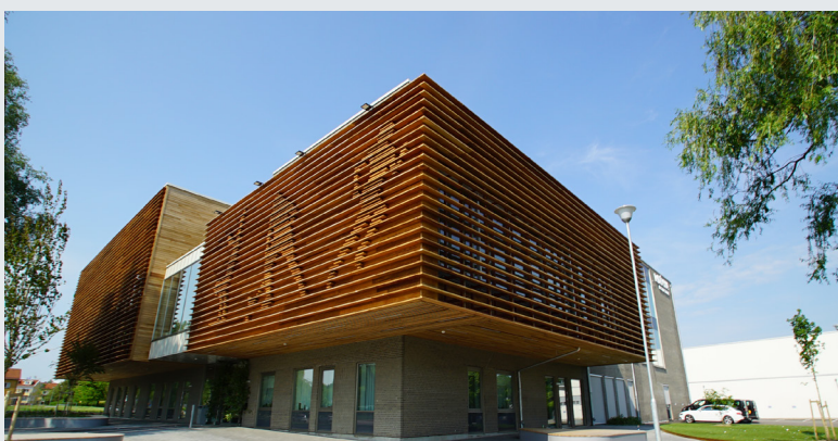
Facts: WRC panels impregnated with Woodsafe Exterior WFX for natural aging with no other surface treatment required.
