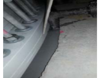
Pumping Masterflow 9400 underneath the flange of the tower
