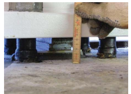
Situation showing tower base installed on shims
