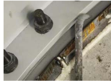
Rigid thin wall metal tube to pump underneath flange
