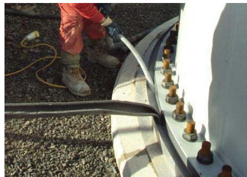
PU-foam used as temporary form
