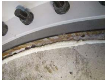
Pumping Masterflow 9400 underneath the flange of the tower
