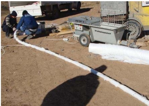
Reflective installation being applied to the hoses
