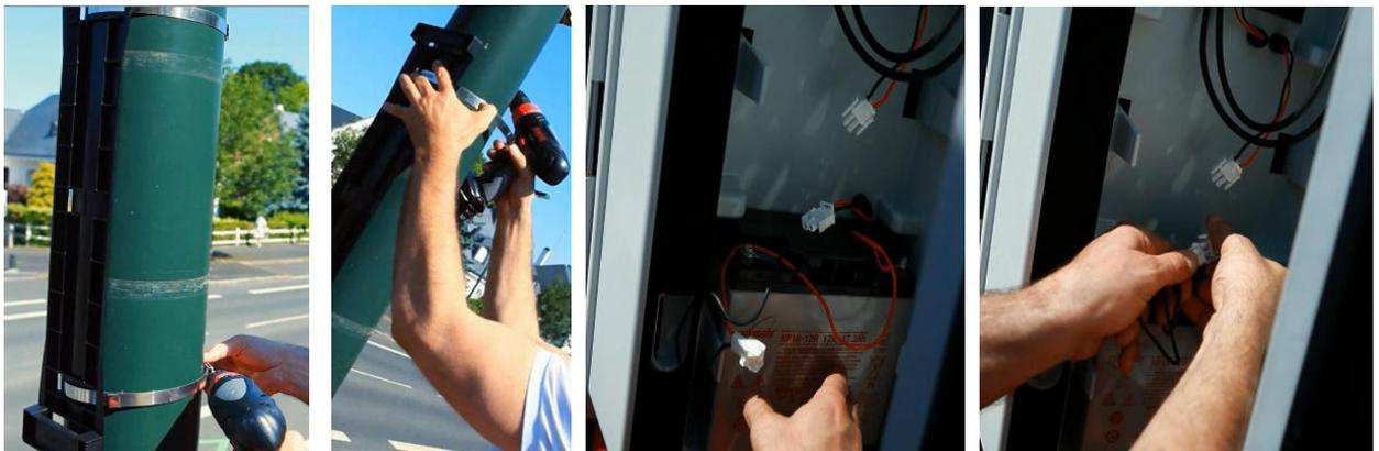
In case of solar power, it is necessary to install the solar panel with its mounting kit before installing the speed sign (**See Solar Panel user guide**)
