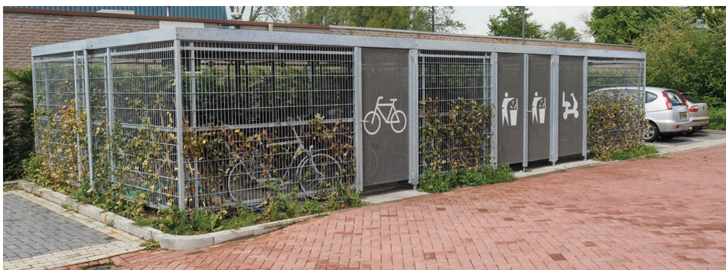
Frame clad with welded mesh and doors clad with perforated steel incorporating distinctive icons - 'bicycle', 'litter' and 'scooters'.
