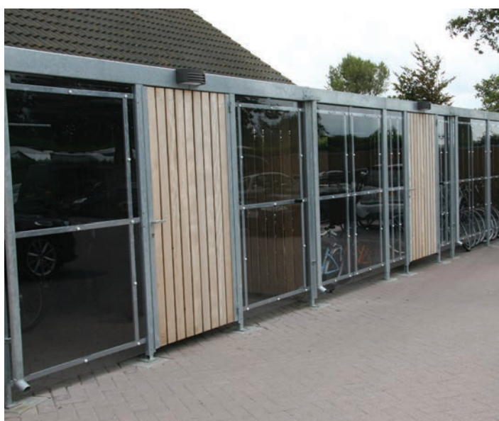
Side walls, back wall and doors frame clad with hardwood. Front wall frame clad with polycarbonate.
