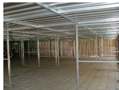
Roof sheets manufactured from corrugated aluzinc sheets
