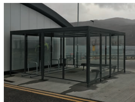
Frame clad with toughened glass
