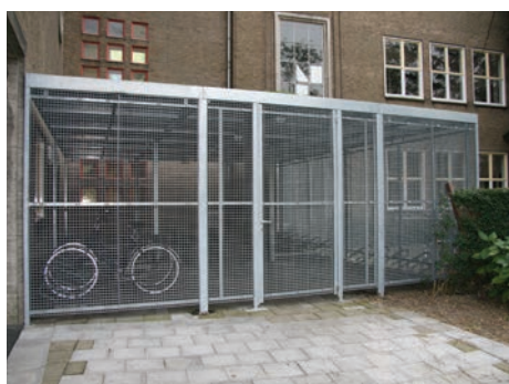
Frame clad with steel mesh
