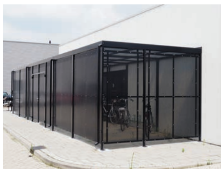
Frame clad with perforated steel and powder coated
