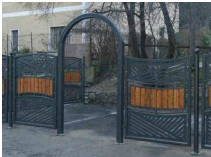
Structure for ecology point made up of closing panel with modular system. Each module is made up of a steel frame in square tube and panel with steel sheet laser cut with decorative part in the middle in pine wooden slats. The lateral supports with decorative sphere on the top can be fixed by ingrounding or at the surface with base plate.
