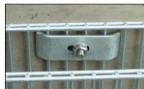
view to rear side threaded rod with single anchor plate
