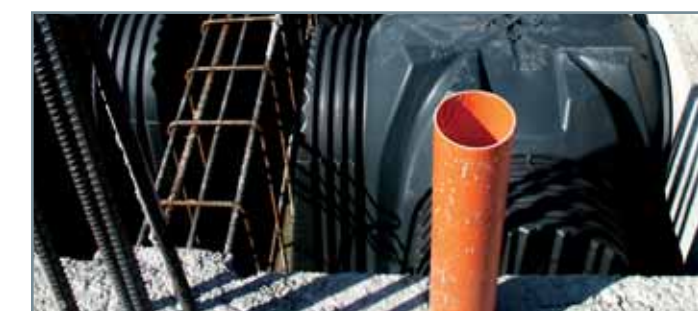
Example of aired foundation with reinforced sub-grade
